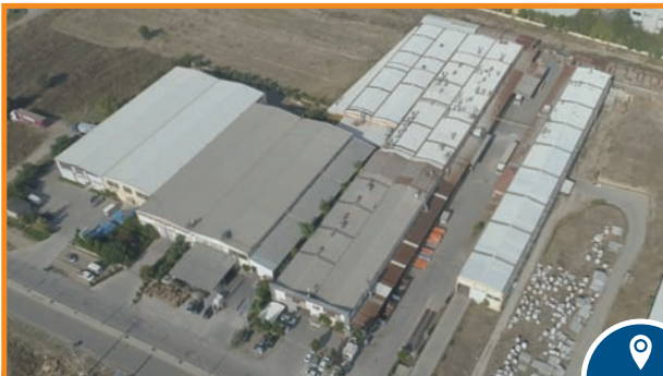
Radiators and Flexo Production
